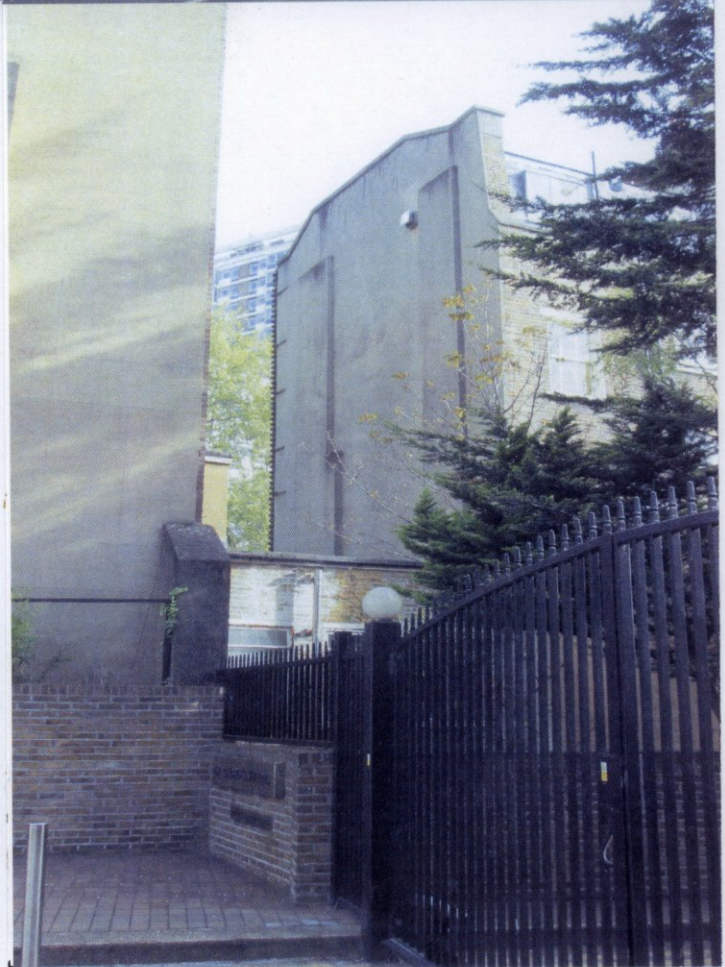
59 Connaught Street front elevation looking west (top) and rear elevation taken from Albion Street (bottom)
